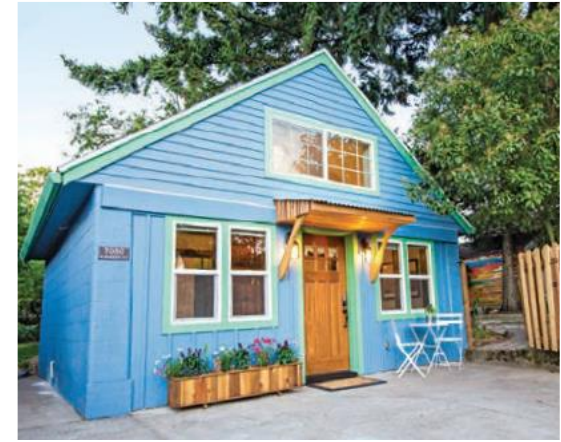
Garage Conversion ADU
